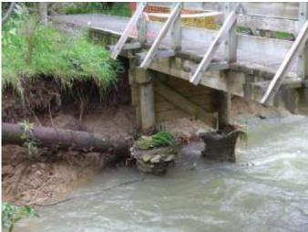
WCC will replace the afflicted bridge 3 early in 2017. The debris trap has been cleared. During the November flood two rock gabions upstream of the debris trap were undermined and fell into the stream. A third gabion slumped. The stream changed course and is jeopardising more gabions. Some of Sathya Sai's plantings opposite were carried away. For Bill Hester's
